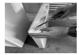
10. Slide the door onto the bottom hinge pin and reinstall the center hinge on the left side (after removing the small stickers and the screw cover that hides the holes).
