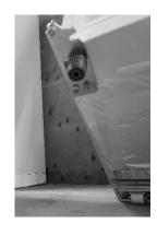
NB: Do not screw all the way in, as these screws are used to adjust the doors.
